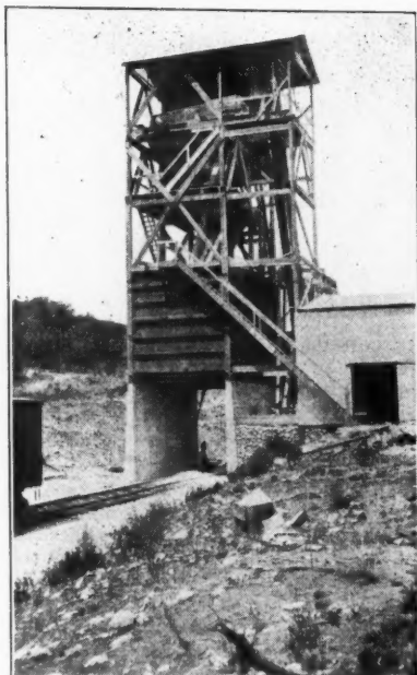
A Close-Up of the Crushing, Screening and Storage Building. This Illustrates the Simplicity of Construction and the Economical Investment
